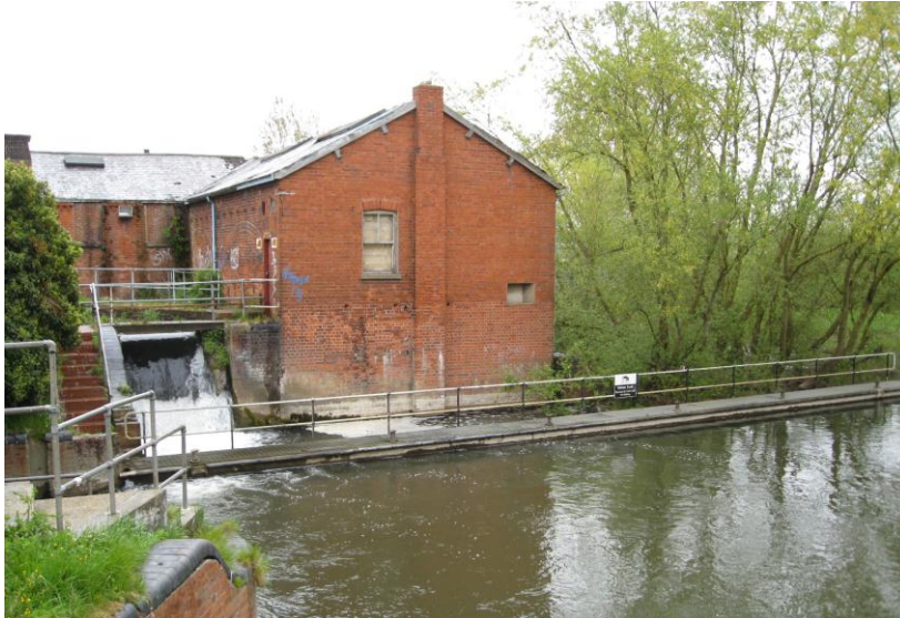
Figure 10 - Example of an impounding structure at Fobney pumping station. Structures like these prevent fish passage and the impounded water results in sedimentation upstream.
