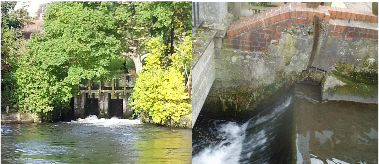
Figure 3 - Examples of physical modifications to the River Kennet, a legacy from historic water mills, which both prevent fish movement and cause impoundment in the upstream reach.
