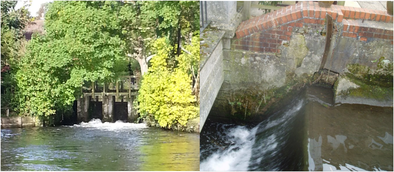
Figure 3 - Examples of physical modifications to the River Kennet, a legacy from historic water mills, which both prevent fish movement and cause impoundment in the upstream reach. These two structures have been modified or bypassed to enable fish passage and improve river morphology as a result of actions in the Kennet Catchment Management Plan and funding from the River Improvement and Catchment Restoration Funds.
