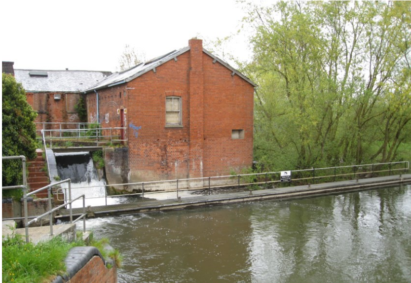
Figure 9 - Example of an impounding structure at Fobney pumping station. Structures like these prevent fish passage and the impounded water results in sedimentation upstream.
